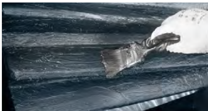
A layer of lubricant must be applied evenly and without air bubbles.
